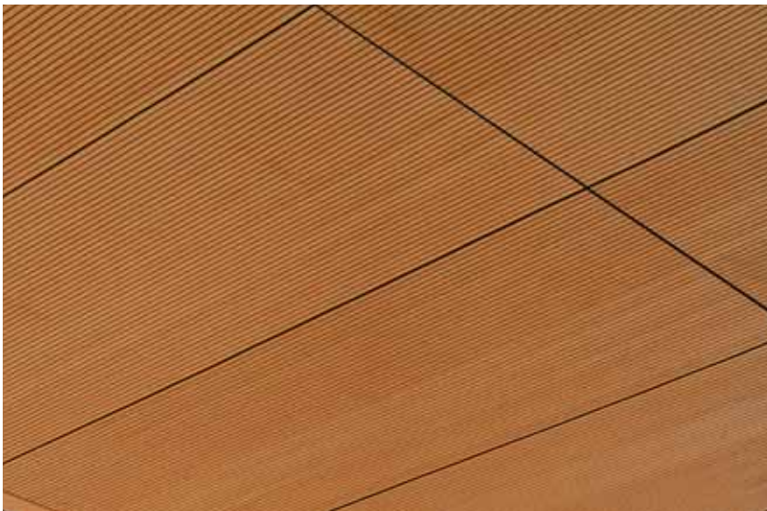
Fully grooved Solo-M panels with quarter cut slipped matched maple veneer. The panels are installed with direct mount hardware onto contractor supplied suspension.
