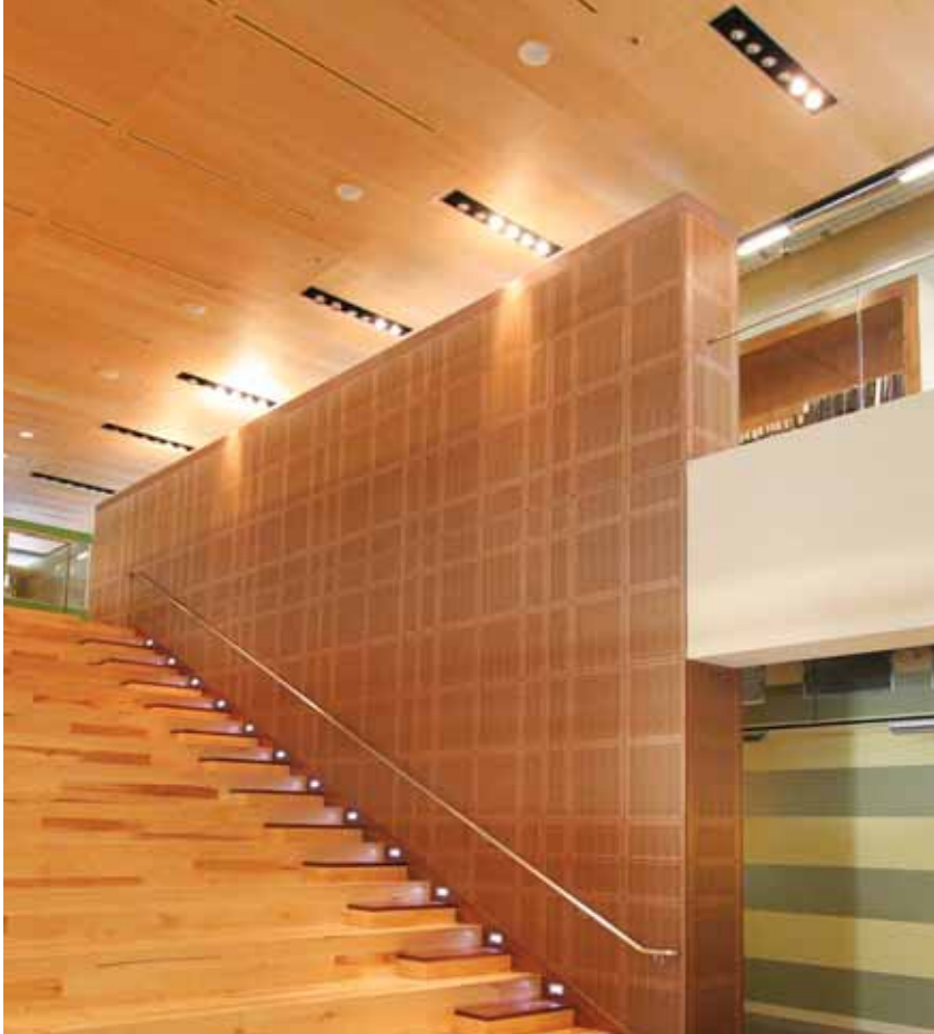
Stop grooved Solo-M wall panels designed with a custom grooved layout and simulated panel joints creating a unique visual appearance.
